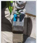
It is essential that the blocks are laid accurately, true to level (±1mm) and vertical (many builders use a simple laser level for speed and accuracy).
