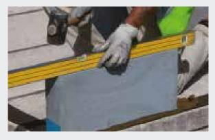
The perpend joints on the first course should be made with Celfix mortar, giving a more rigid base in a shorter time.
